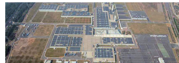
Solar panels at GTMC
